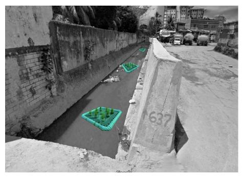
Figure 2.19. Recommended spacing for the constructed floating wetland.
